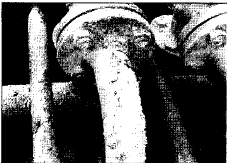
Fig. 1 Corrosion defects on the steam pipe of ship
