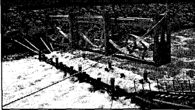
Fig. 1 Tidal current power plant in the Hadong power plant
