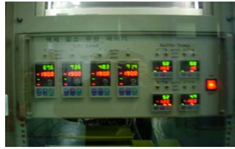
Picture 1. The front view of the LN_2 controlling module.
