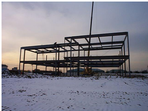
Figure 4. Steel frame under construction
