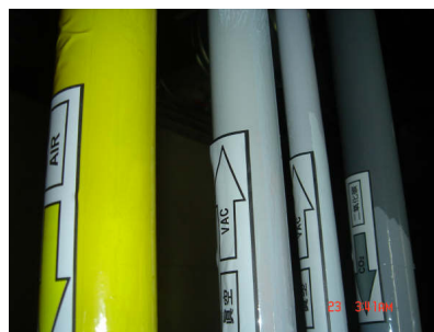
Figure 6. Pipes with clear color and tags
