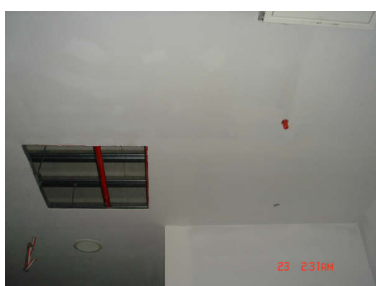
Figure 4. Gypsum board with epoxy paint ceiling
