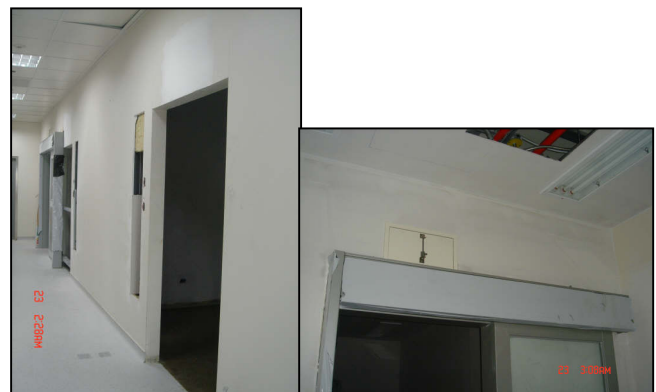
Figure 3. Washable and easily cleaned surface and perfect junctions with ceiling
