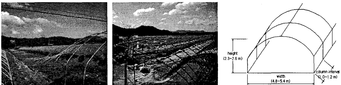
Fig. 1. Case of damaged single-span greenhouse at Sungju area
