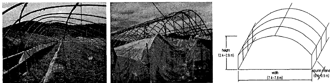
Fig. 3. Case of damaged single-span greenhouse at Goryeong area
