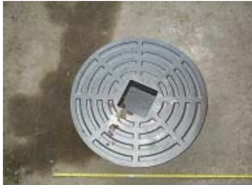
(c) the cover of a manhole
