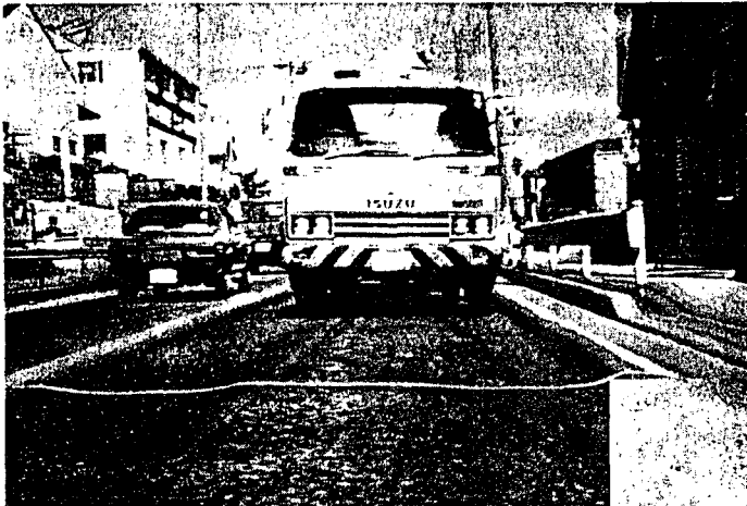
Fig.1-1 Example of Heavy rutting (ex.RD \geq 30m m) < in Japan >
