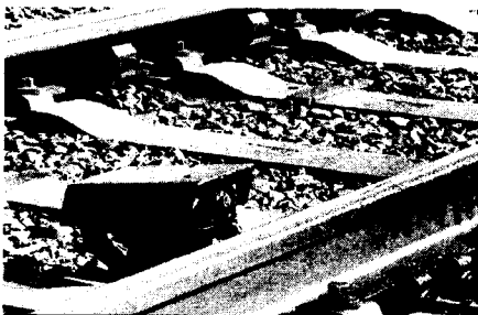
Fig. 5 Rail lubricator(side of rail)
