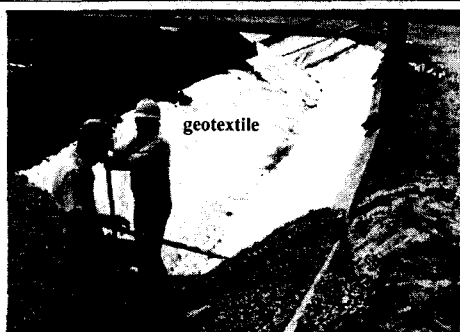
Trench in construction: separation
