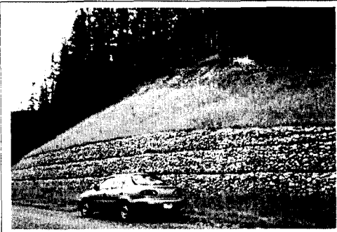
Reinforced wall with GTX and gabions
