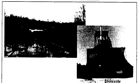
An access road: reinforcement
