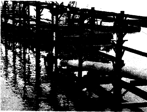
Fig. 10 Pulling head arrangement
