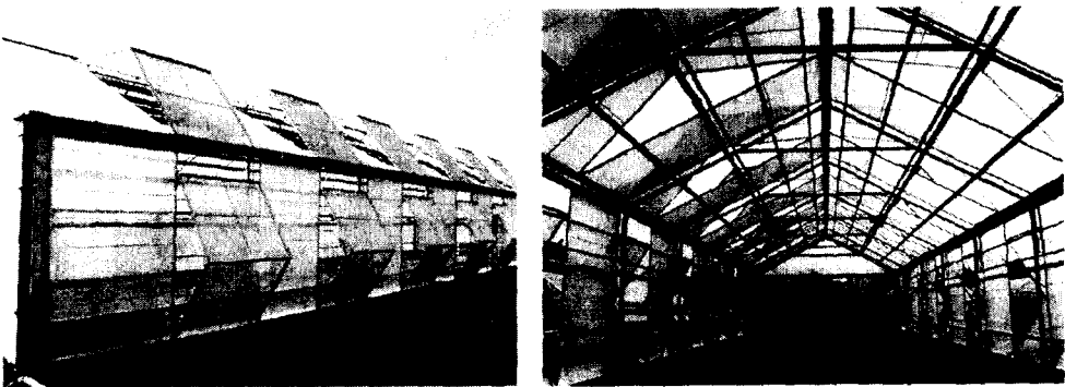
Fig.2. Model greenhouse consisted of bending panel type windows
