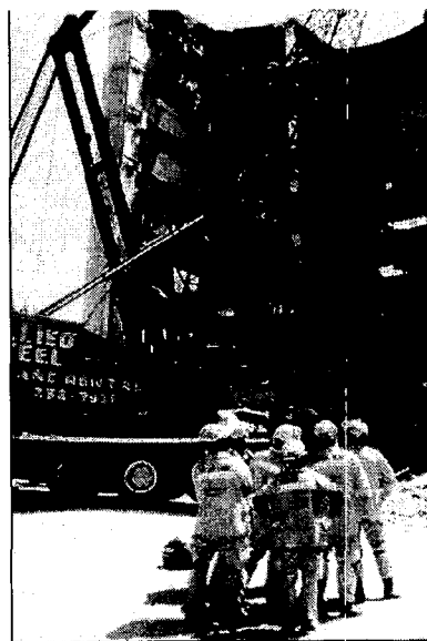
Figure 4. Urban Search And Rescue Team Survey The Murrah Building Site. (FEMA News Photo).
