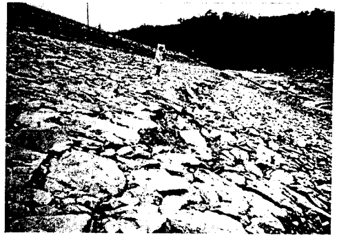
Photo 3. Kitayama Dam No. 1 : Shallow sliding at the upstream slope.
