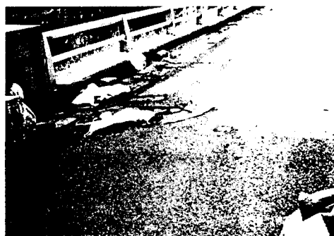
Photo 2. Tokiwa Dam : Cracking at the crest.
