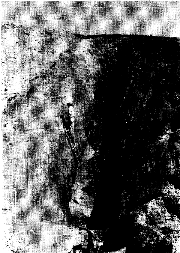
Fig.2 Trench work with the size of 25m in length, 4m in depth and 5m in width at Kalgok-ri, Cheonbuk-myeon.
