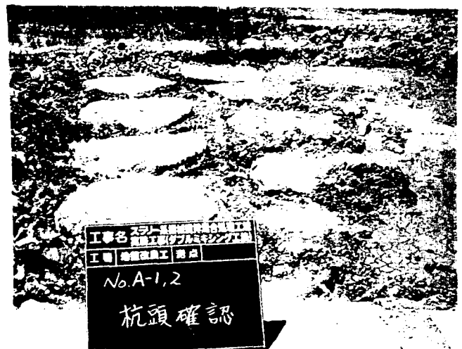
Photo 1 Soil-cement columns after construction
