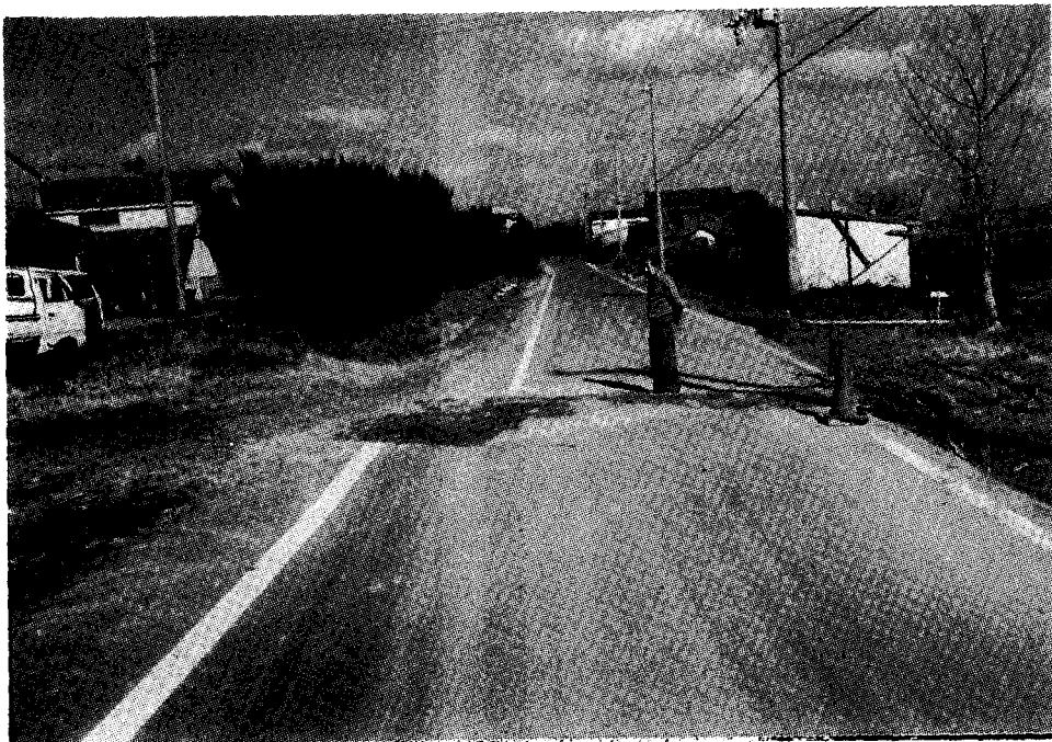
Fig.2 Displacement of road about 1.5m along the fault in Awazi island.
