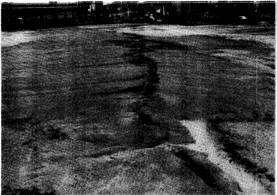
Fig.4 A zone of mud boils on the ground in Port-island.
