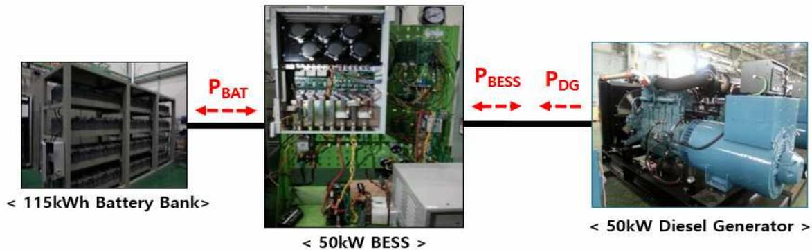
Fig. 15. Hardware configuration of BESS and diesel generator in the stand-alone microgrid
