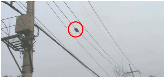
Fig. 7. Field test for overhead distribution power lines.
