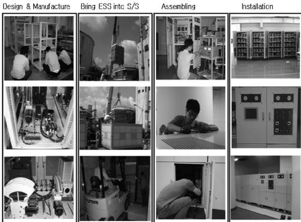
Fig. 2 Developing and installing process
