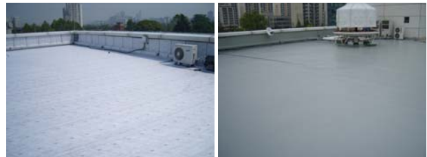
(a)Waterproofing layer installation (b)Root barrier sheet installation
