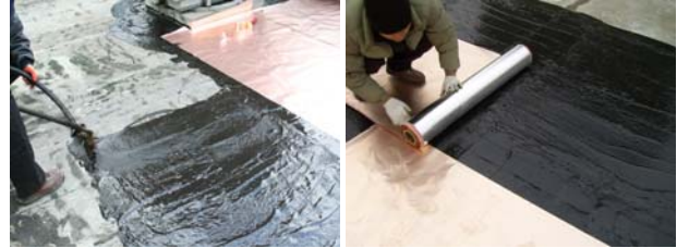
(a)Waterproofing layer installation (b)Root barrier sheet installation
