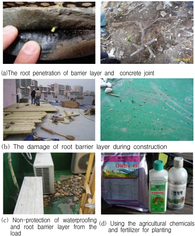
Figure 1. Construction and maintenance situations of the green roof system
