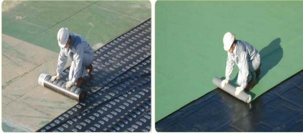
(a)Waterproofing layer installation (b)Root barrier sheet installation
