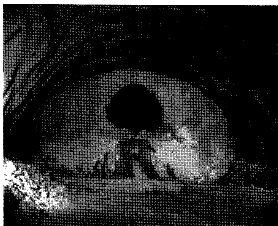
Photo 1. Photograph of cutting face of the actual tunnel.
